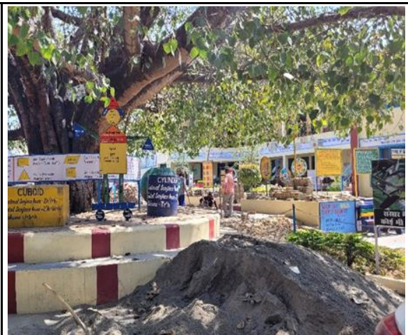
Ongoing construction work at SoE, Badhani, Pathankot
