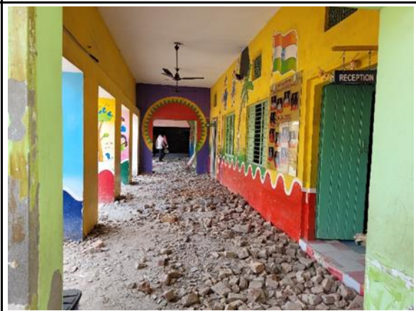
Ongoing construction at Government Smart Primary School, Chananwala, Fazilka
