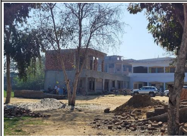
Ongoing construction at Govt. Elementary School, Khadur Sahib, Taran Taran
