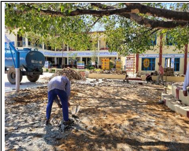
Ongoing construction work at SoE, Badhani, Pathankot
